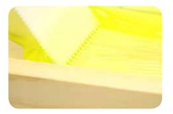
Measure and mix the resin and hardener before pouring out the mixture in one go and if required using a spreader to ensure full coverage. Don't forget to double pot the mixture.
